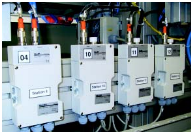
Assembly line for jalousie modules at Henkel + Roth GmbH
